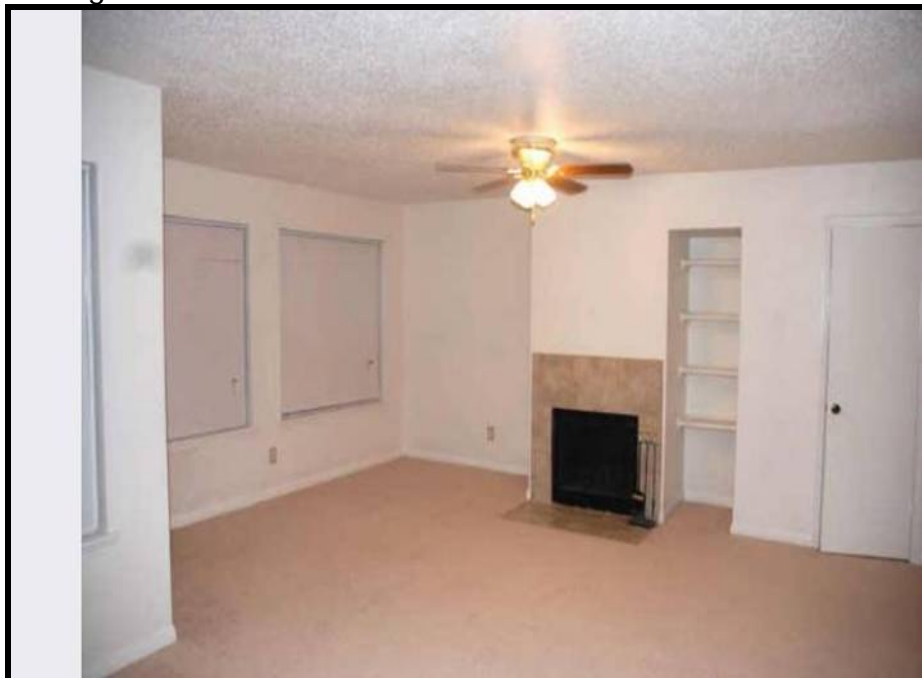
Living Room Pre Renovation
